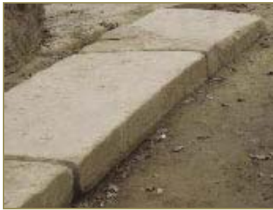
SANDSTONE PLATES ON W SIDE
