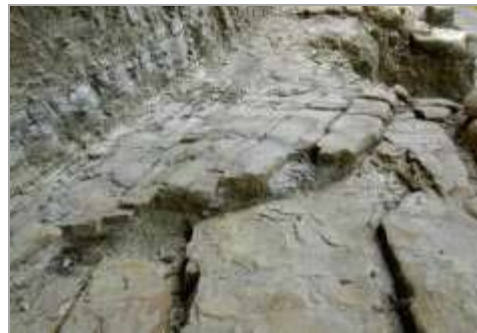
WORN-OUT TILES ON A ROCK TERRACE
