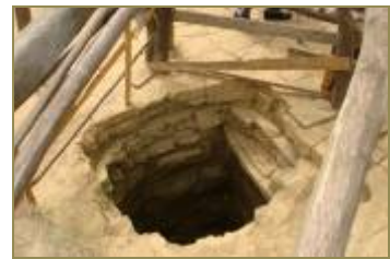
A HEAVY STONE STRUCTURE WITH AN INCLINED SURFACE. ABOVE IT ARE TWO TERRACES, SEEN IN SECTION. A WELL SUNKEN FOR A FEW METERS SHOWS MULTI COURSES OR LAYERS OF STONE.
