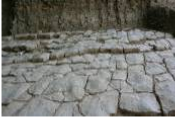
At SB 12, well preserved tiles
